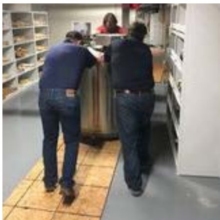
Left F5: Each tank was carefully moved to its new location in LN room. The floor was protected with plywood.
